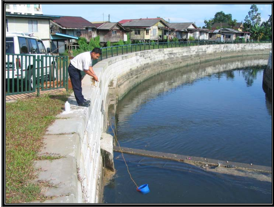
Fig. 7 Progress Photos Taken In December, 2006
