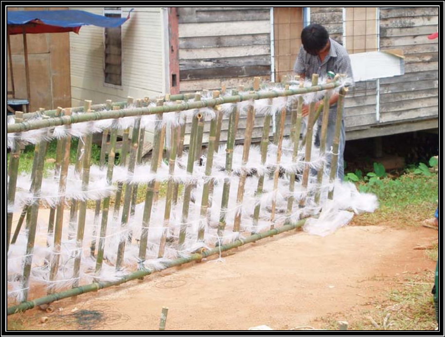
Fig. 5 Biomedia Frame under construction
