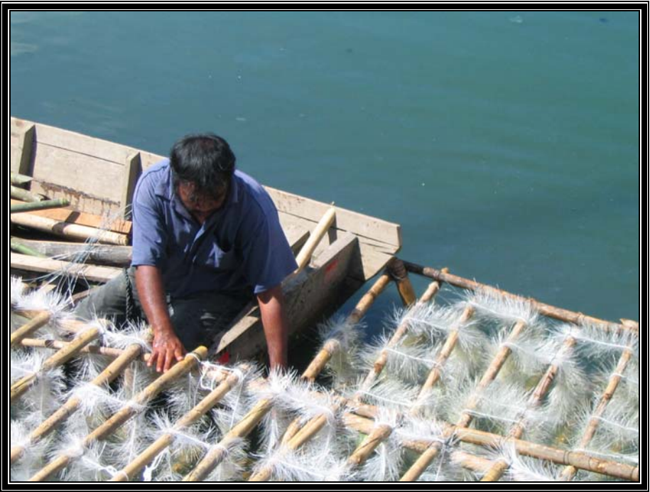
Fig. 6 Installation Of Biomedia
